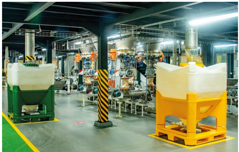
New Spice plant facility.
